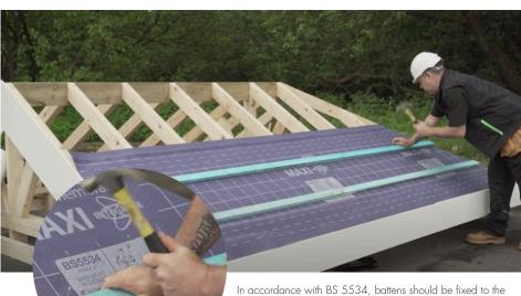
In accordance with BS 5534, battens should be fixed to the rafters at centres of no more than 600mm apart, using nails that provide a minimum of 40mm penetration into the rafter. To achieve this a nail length of 65mm is recommended.
