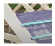
Starting at the lower edge of the roof, nail the battens into place directly into the rafter centres. Each batten should overhang at the verge by 30- 50mm to allow the correct installation of the verge units.
