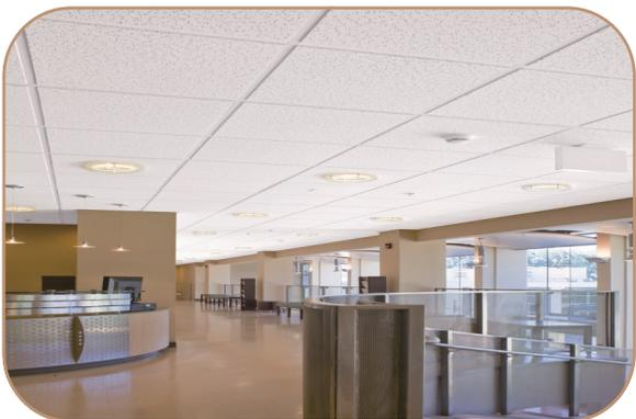
Armstrong suspended ceilings are designed for maximum effect with modest cost and fast installation times. The professional steel framing interlocks for rigidity and is fully Fire Rated for areas with public access. An easy to assemble system that gives you a neat and clean finish to any ceiling.
