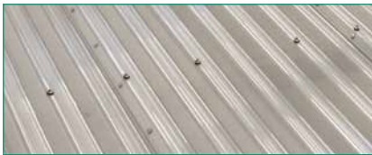
2 Primary Fixing at every other corrugation
