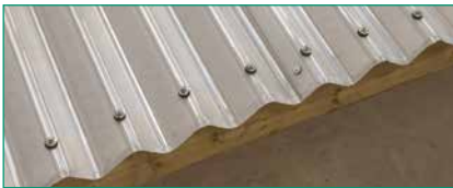
1 Primary Fixing at every corrugation
